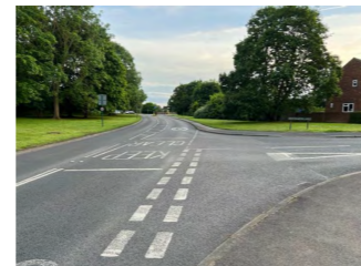
Above: wide, sweeping radii break pedestrian and cycle desire lines; increase vehicle speeds whilst also making them difficult to cross. Off site improvements could reconfigure the radii on this junction as part of a development to village centre series of improvements.
